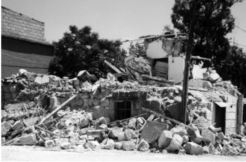
Figure 5. Collapse of older residential structures at the village Misis.
